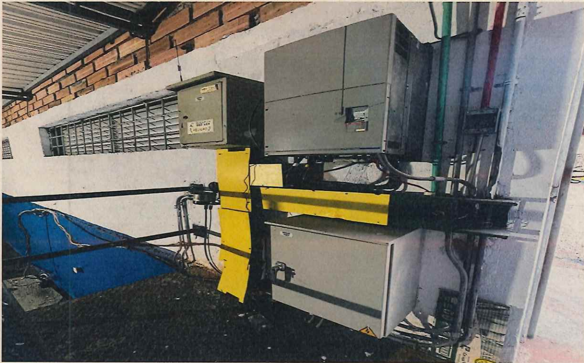
EBAR BOULEVARD DEL RIO
